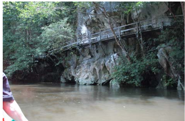
Boardwalk engineering on the way to Clearwater Cave
